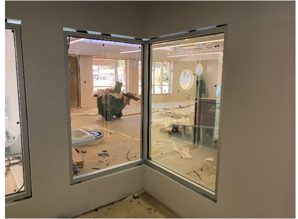
Observation room glass installed at the YMCA
