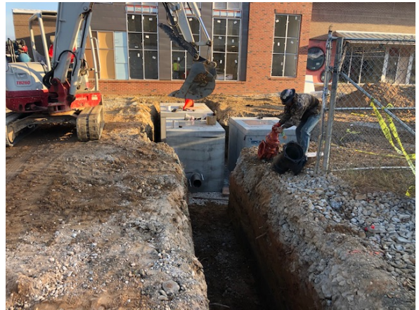
Water vaults set at YMCA
